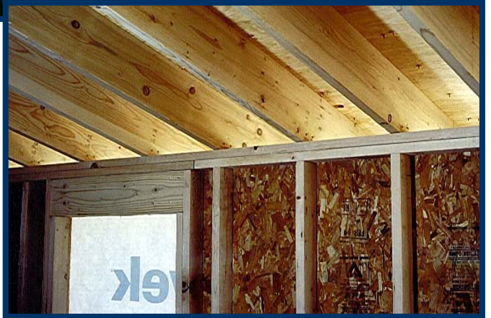
A Utility Building during Construction
