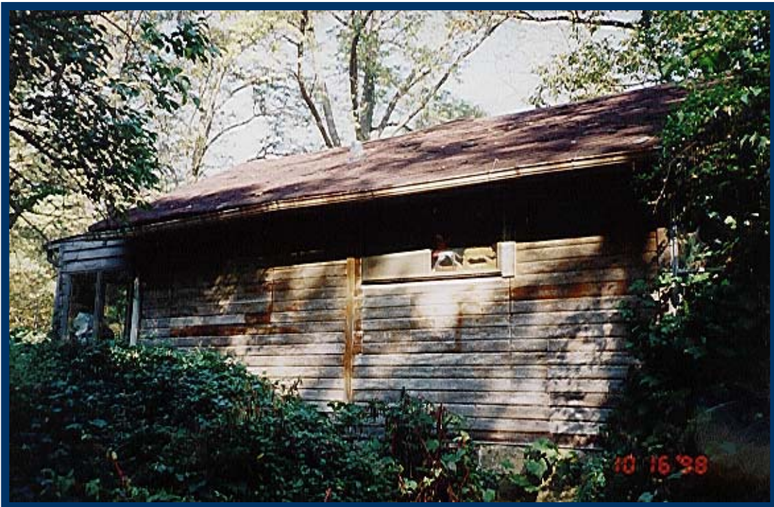
Exterior of Home Awaiting a Paint Covering
